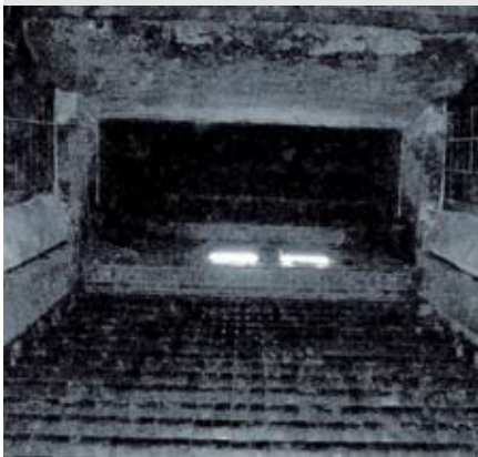
Grate bars in waste incineration
